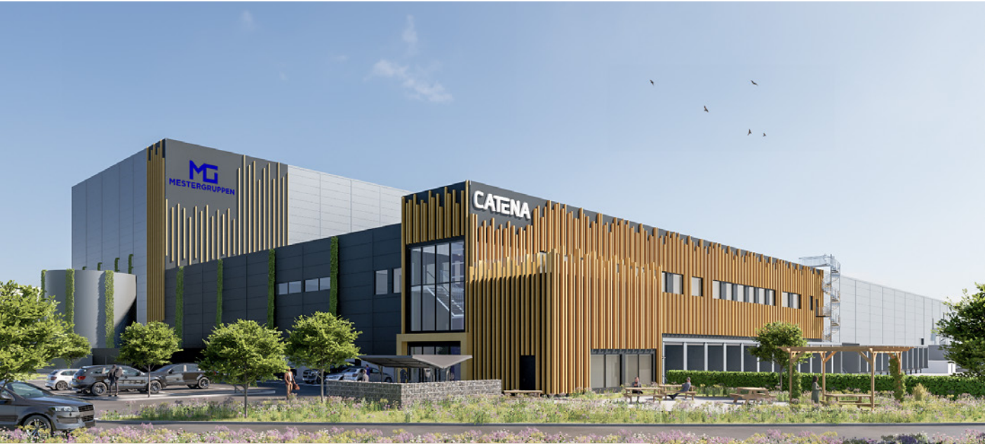
Mestergruppen's new logistics centre in Jönköping, which achieved BREEAM Outstanding certification.
